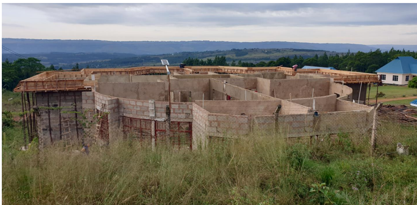
Photo no 7: MHOLA Rehabilitation Facility for children with special needs - Construction on progress
